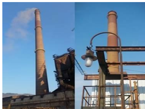
Sinter plant stack before and after installation of the filter
